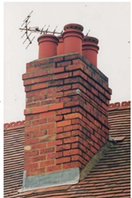
*Watch out for blocked or removed flues—are these vent caps placed on live flues?*
