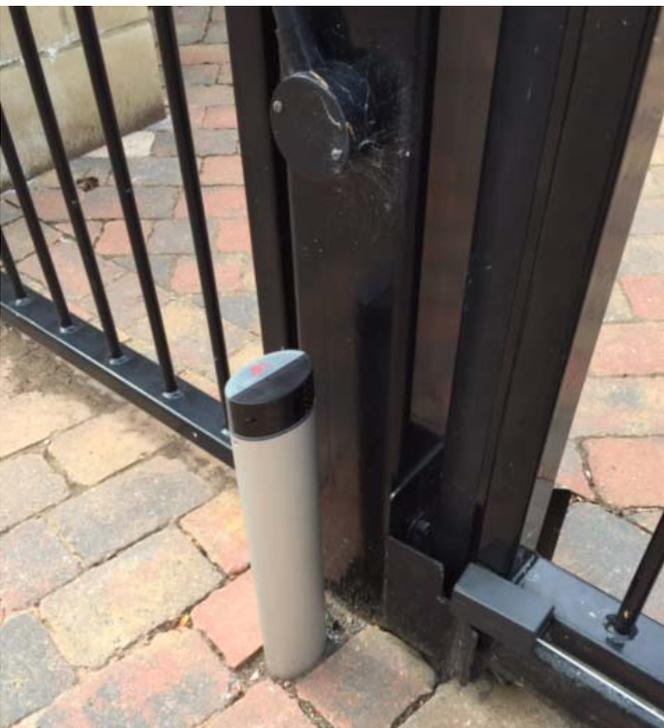
This is one half of the light beam across the opening. When the gate was shutting, I walked through the beam, the gate stopped and then opened.
